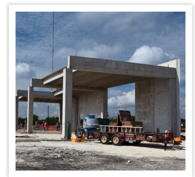
Purpose-built data center under construction
